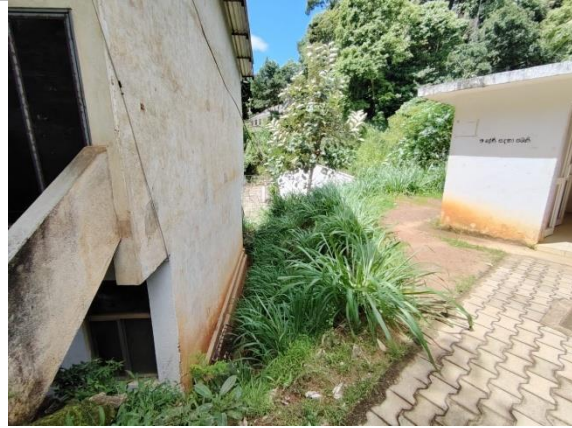
Figure 4a: Mitigation location of Wariyapola Sri Sumangala College, behind Grade 9 building (Location 1)
