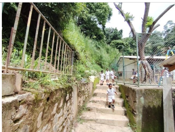
Figure 4f: Fence, retaining wall and stair case adjacent play area and Grade 1 (Location 2)
