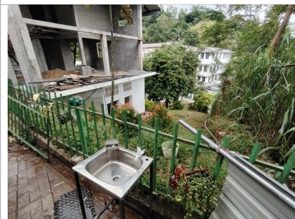
Figure 4i: Fence and water line adjacent to the boundary of Sumangala College and Sylvester's College. Three storey building (Under construction) is nearby the mitigation location and the school boundary (Location 3)
