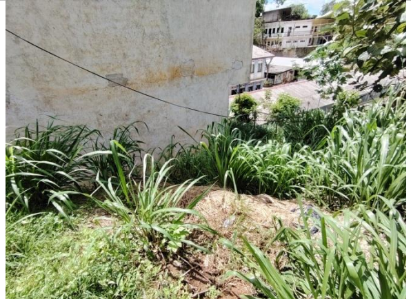
Figure 4b: Approximately 4m high slope with 70° inclination and Electricity line along the slope section (Location 1)
