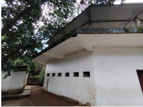
Figure 4k: Pavilion and Music room of two storey building adjacent to the playground, and washroom near by the mitigation area (Location 3)
