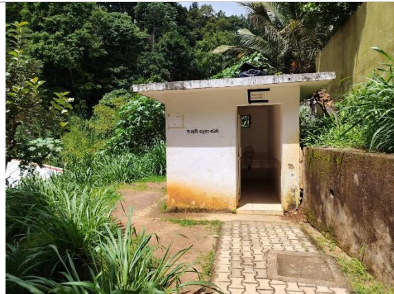
Figure 4c: Washroom and retaining wall nearby the mitigation location (Location 1)
