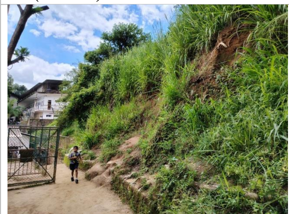
Figure 4e: The toe of the upslope area with retaining wall, vegetation and soil erosion adjacent to the play area (Location 2)
