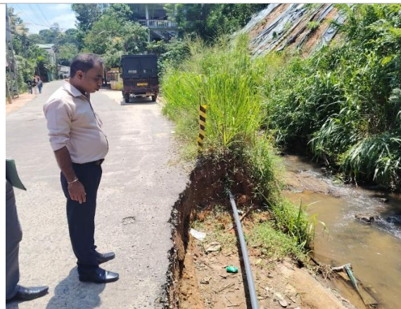
Figure 4c: Water stream flow along Kiribathkumbura – Wathurakumbura road near to the mitigation location 01 (L1)
