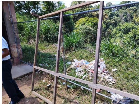
Figure 4d: Fence net near by the edge of the slope at the location 02 (L2)
