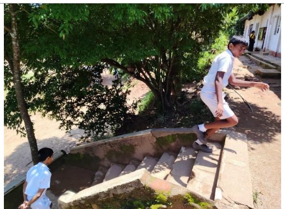
Figure 4j: Staircase nearby the location 02 which provide access to the Martin Wickramasinghe building (L2)
