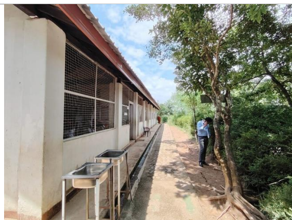
Figure 4l: Downslope in front of the Ediriweera Sarathchandra building (single storey) at location 03 (L3)
