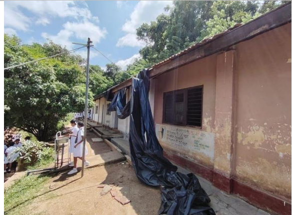
Figure 4f: Wash basin and water line nearby the location 02 (L2)
