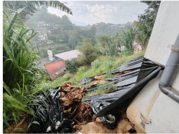
Figure 4g: Soil mass failure and soil erosion adjacent to the Grade 6, 7, and 8 building (Location 2)
