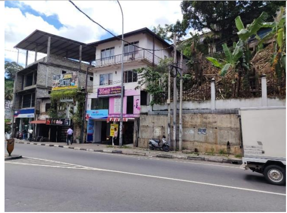
Figure 4m: Three-storey private building adjacent to mitigation Location 03, retaining wall and the Kandy - Jaffna main road (A9)
