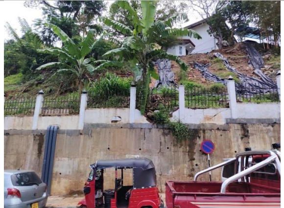
Figure 4n: Steep slope of Location 03 with vegetation and school boundary
