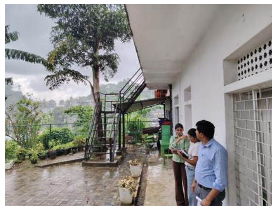
Figure 4d: Affected two-storey building with staircase and fence net (Location 2)
