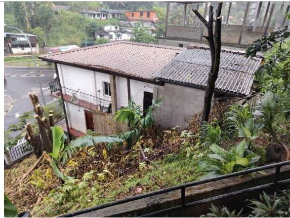
Figure 4g: Soil mass failure and soil erosion adjacent to the Grade 6, 7, and 8 building (Location 2)
