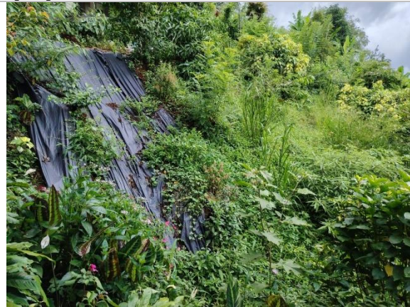
Figure 4c: Location 1; Unstable areas covered with polythene layers
