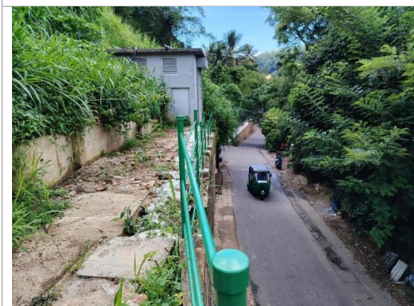
Figure 4i: Location 4 ; Transformer room, Boundary wall, fence and the access road
