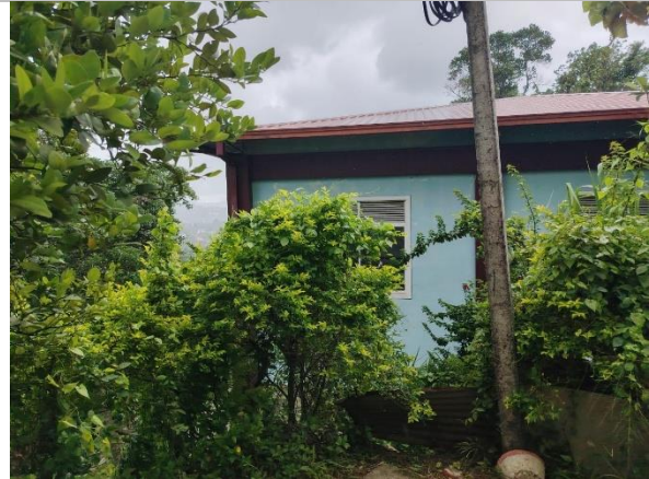
Figure 4l:Location 4; Grade 8 and 9 classroom building
