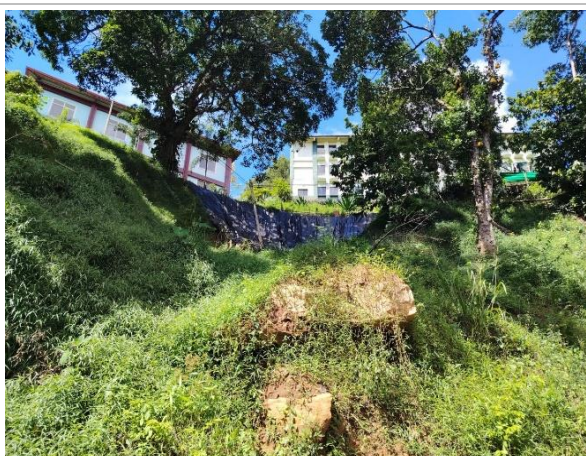
Figure 4b: Location 1; Upslope area of the access road
