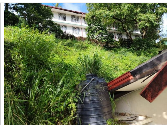
Figure 4p: Location 7; unstable slope located behind the dental center building
