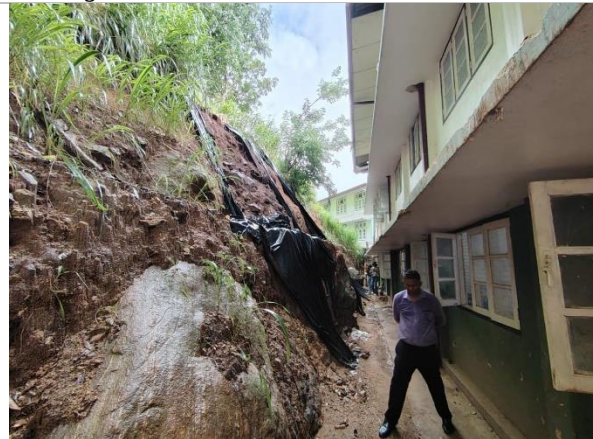
Figure 4n:Location 6; failed slope located behind the Science Section building
