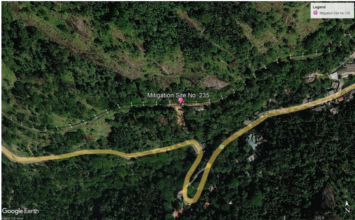
Figure 3c: Google image of the proposed landslide mitigation Site No. 235, the surrounding environmental features and service infrastructure.
