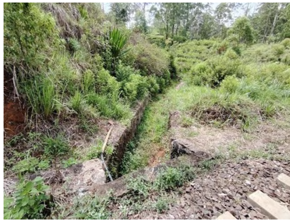
Figure 5i: Culverts, Vegetation of the area and community water supply lines
