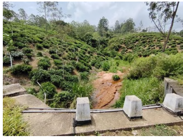
Figure 5d: Seasonal water stream and community water supply lines
