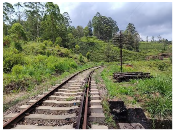
Figure 5b: Electricity line across the railway line from Kotagala to Talawakele
