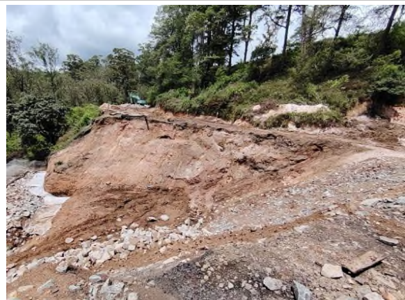
Figure 5c: Vegetation and washed-out railway which is used as access road for commuters
