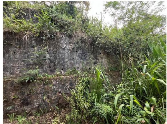
Figure 4b: Retaining wall and the upslope area
