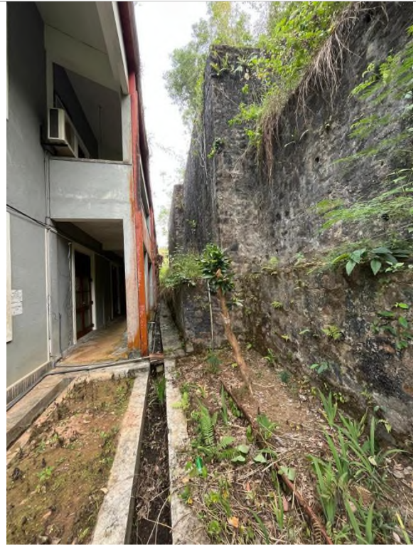
Figure 4h: Retaining wall and drainage behind the court building
