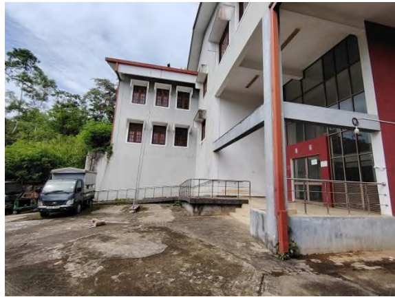
Figure 4a: View of the court complex building
