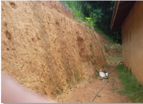
Cut slope in location 01 (behind the grade 07 building)
