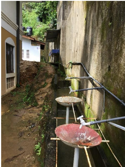
Figure 5c: Water supply line
