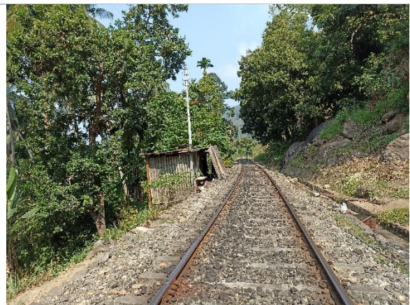
Figure 7d: Railway line
