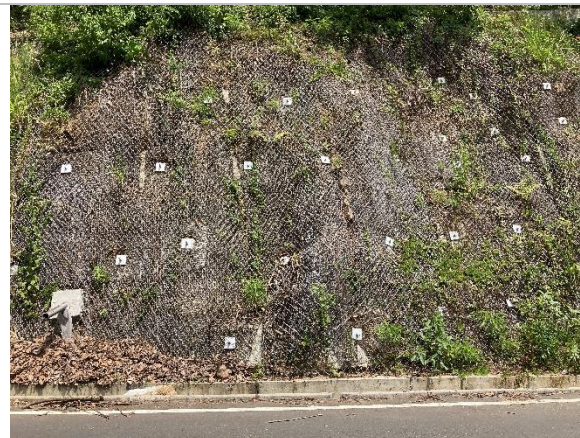
Figure 6e: Existing remedial measures which have already undertaken to reduce the potential risk in upslope area such as netting, soil nailing and horizontal drains
