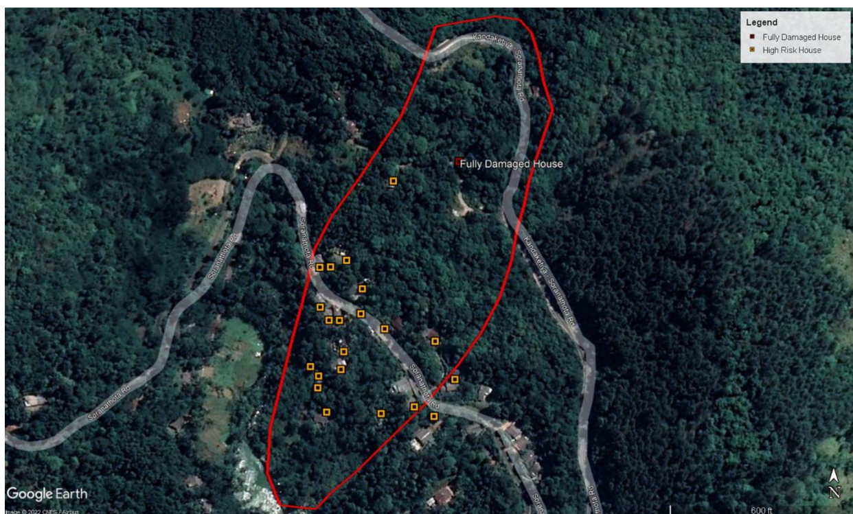
Figure 4: Location of totally damaged house and high-risk houses due to potential landslide
