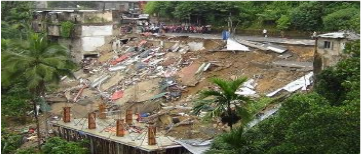
Figure 5: Area after the road failure (Source:Dailymirror on 19.07.2019 )
