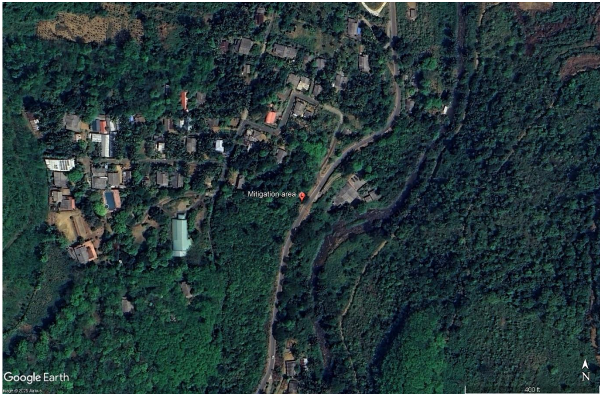
Figure 2: Google image of the proposed rock-fall/ landslide mitigation site, the surrounding environmental features and service infrastructure
