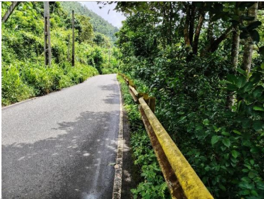
Figure 5e: RHS of the Road section and RDA fence (L3)
