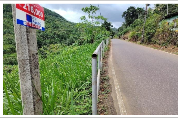
Figure 5w: Safety RDA fence (L8)
