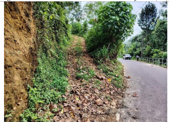
Figure 5m: Access Road to Rubber plantation (L5)
