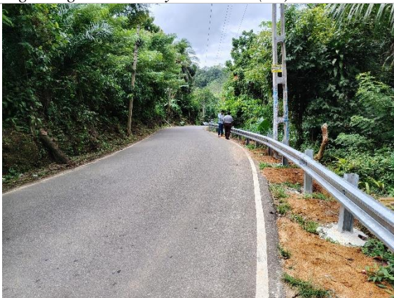
Figure 5i: RHS of the road and RDA fence (L4)
