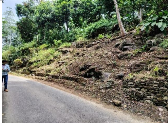
Figure 5c: Up slope of the LHS of the road (L2)
