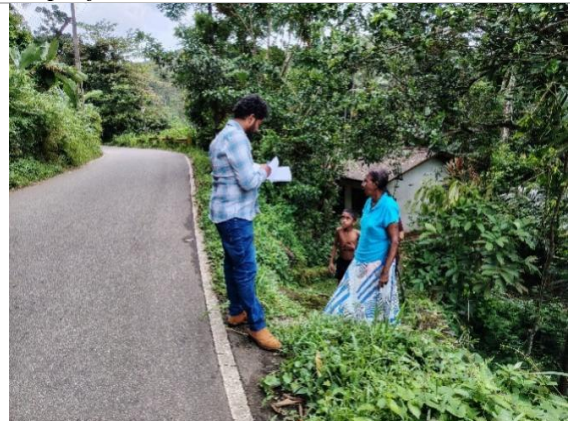
Figure 5b: Failed down slope section (L1)
