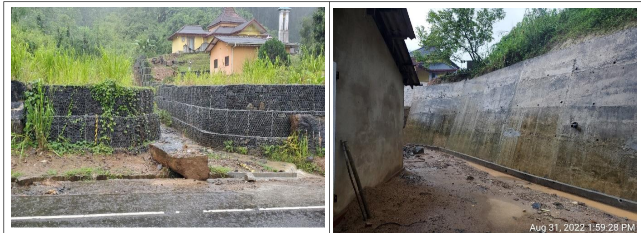
Figure 03. Remediation measures taken after the initial landslide
