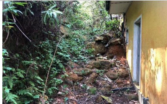
Figure 4b: Fallen rocks and soil debris to the rear side of the building
