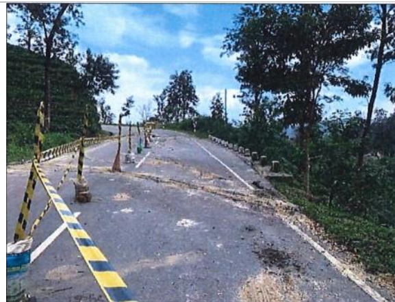
Figure 5c: Damaged road with tensional cracks
