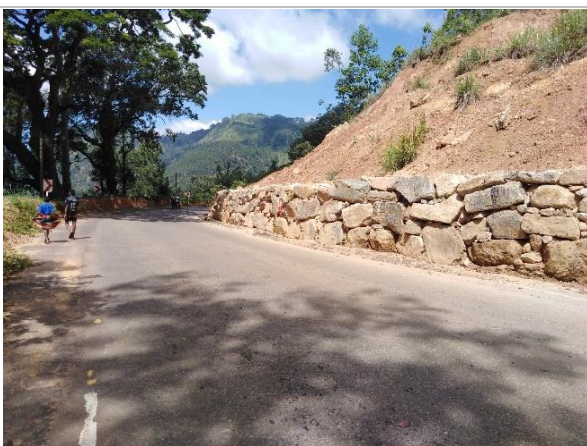
Figure 5e: Temporary built retaining wall
