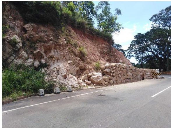
Figure 5a: Slope failure
