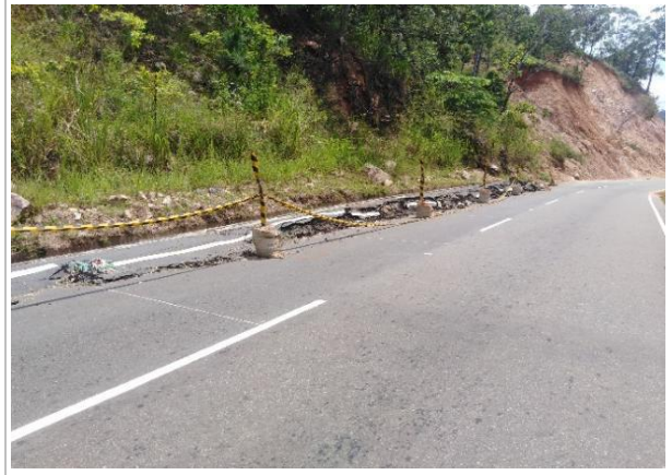
Figure 5b: Uplift road section
