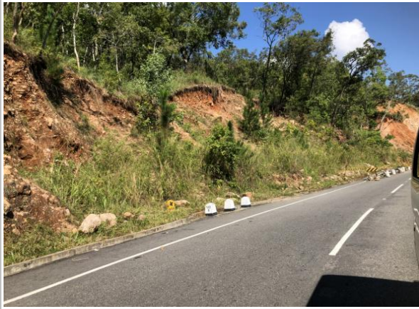
Figure 5a: Up slope failed section with unstable trees
