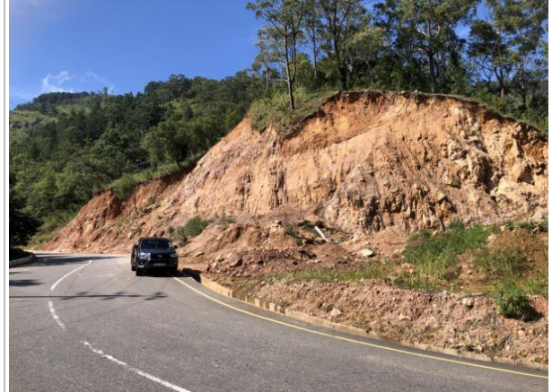
Figure 5d: Up slope failed section with road bend area
