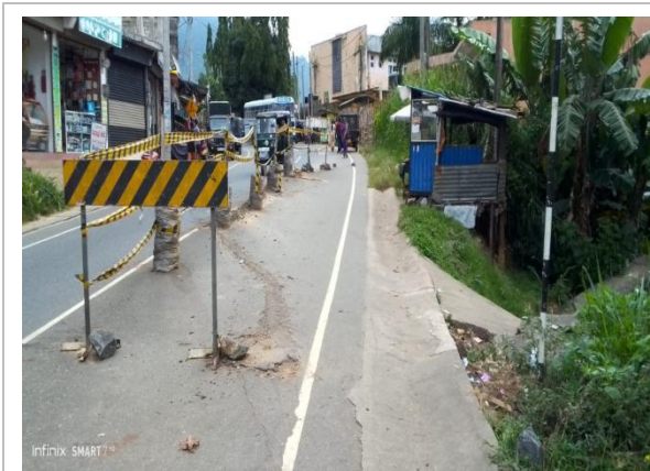
Figure 6a: Damaged road section of Peradeniya-Badulla-Chenkaladi highway (A5) Tension cracks are seen parallel to the road
