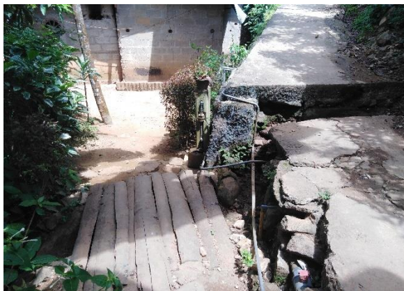
Figure 6e: Damaged access road section and water supply line of Pradeshiya Sabha - Passara
