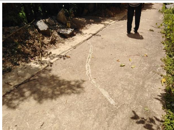
Figure 6h: Cracked concrete road to the down-slope area
