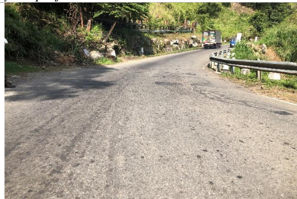
Figure 4b: Cracked and subsidized section of the road
