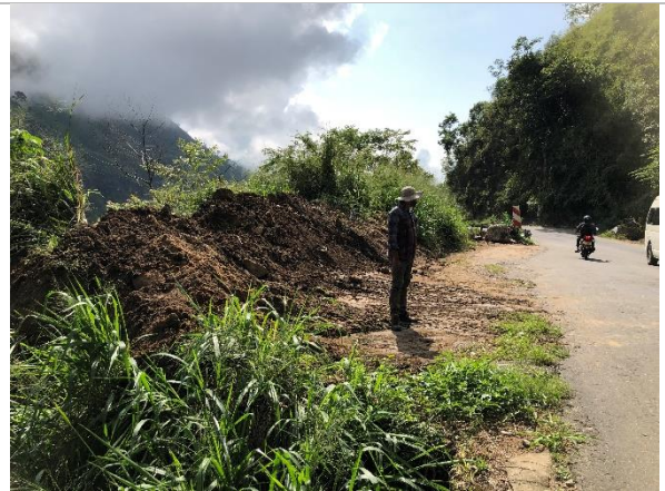
Figure 4d: Rock boulders and soil masses rest at the downslope
