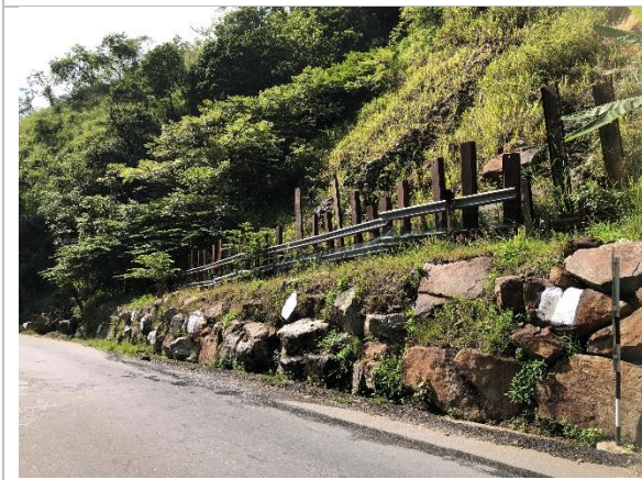
Figure 4e: Temporary constructed metal fence and rubble wall
