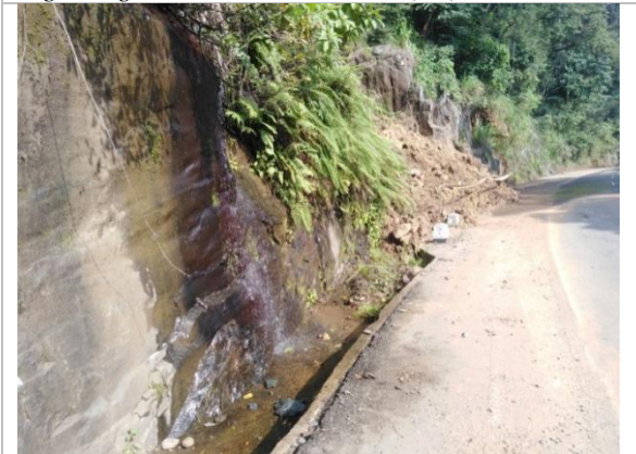
Figure 3i: Water seepage (L3)
