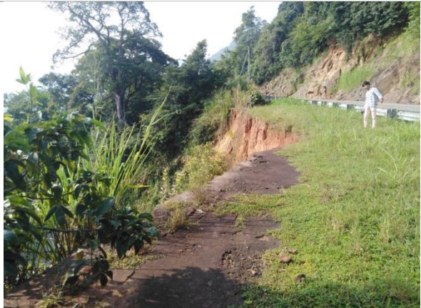
Figure 3b: Failed upslope section (L1)
