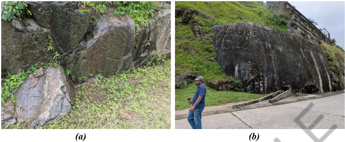
Figure 3.21: (a) Seepage through jointed rocks and; (b) retaining structure for portion of slope at RHS slope of Raja Mawatha (B492)
