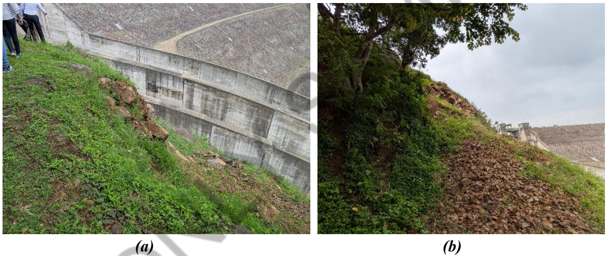
Figure 3.19: (a) Failure at the top berm level and; (b) accumulation of the debris on the bottom berm level of LHS lower slope of the Raja Mawatha (B492) (slope between road and spillway chute)
