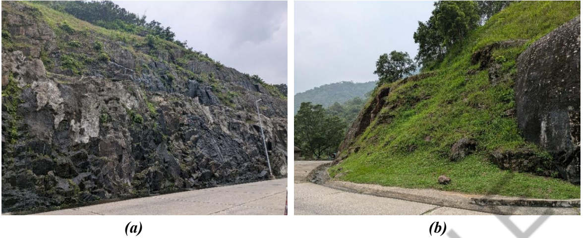
Figure 3.18: (a) Jointed rock slope and; (b) Weak rock band with higher weathering near Randenigala Dam
