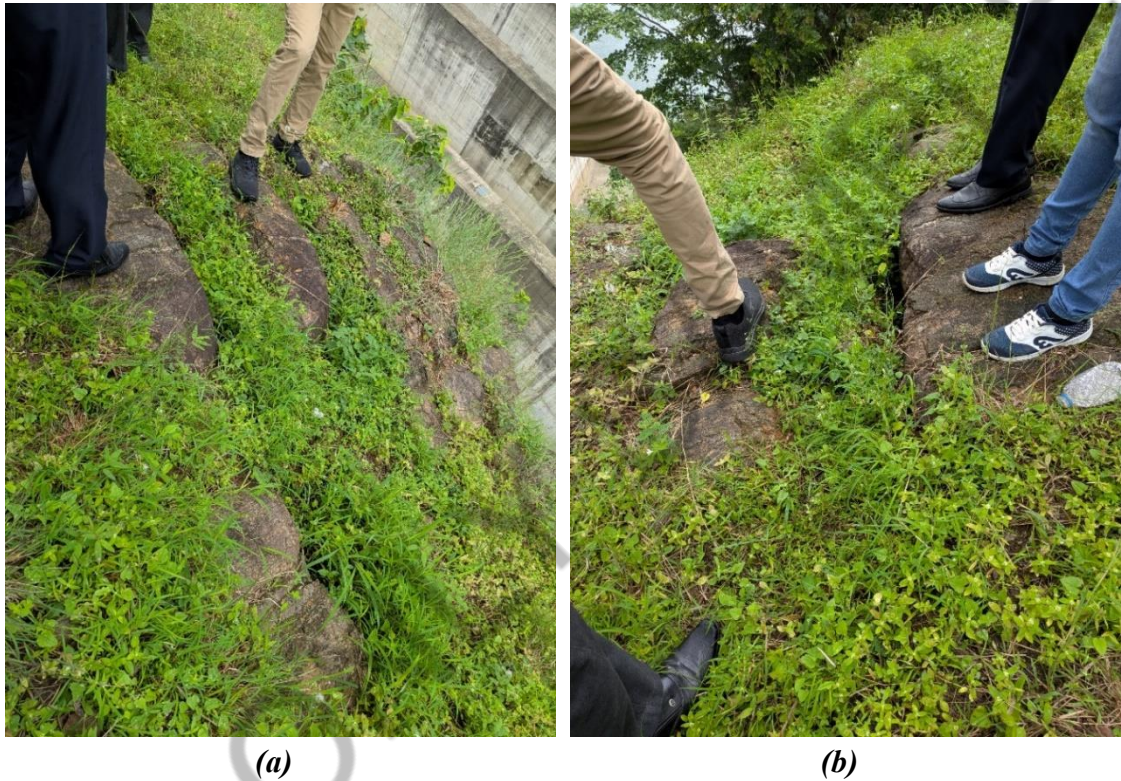
Figure 3.20: (a), (b) Open displacement crack at top berm level of LHS slope of Raja Mawatha (B492)
