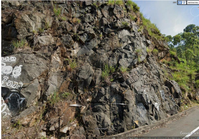
Fig. 3.4 Photograph of the fractured rock slope
