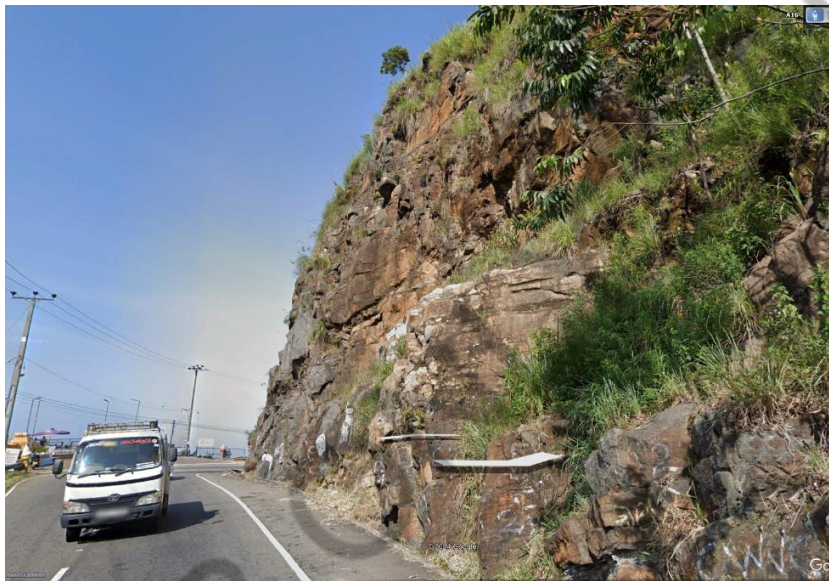
Fig. 3.5 Photograph of the fractured rock slope
