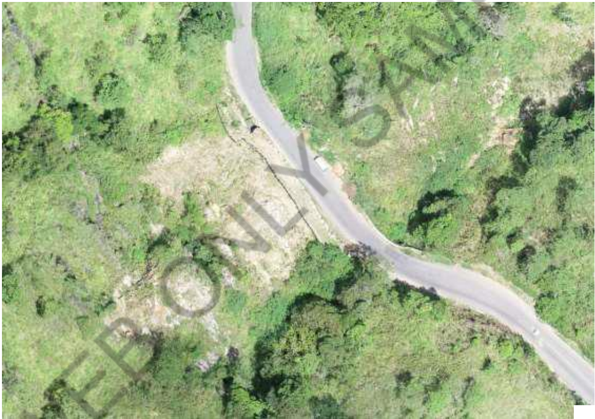
Fig. 3.16 Drone image of the failure location
