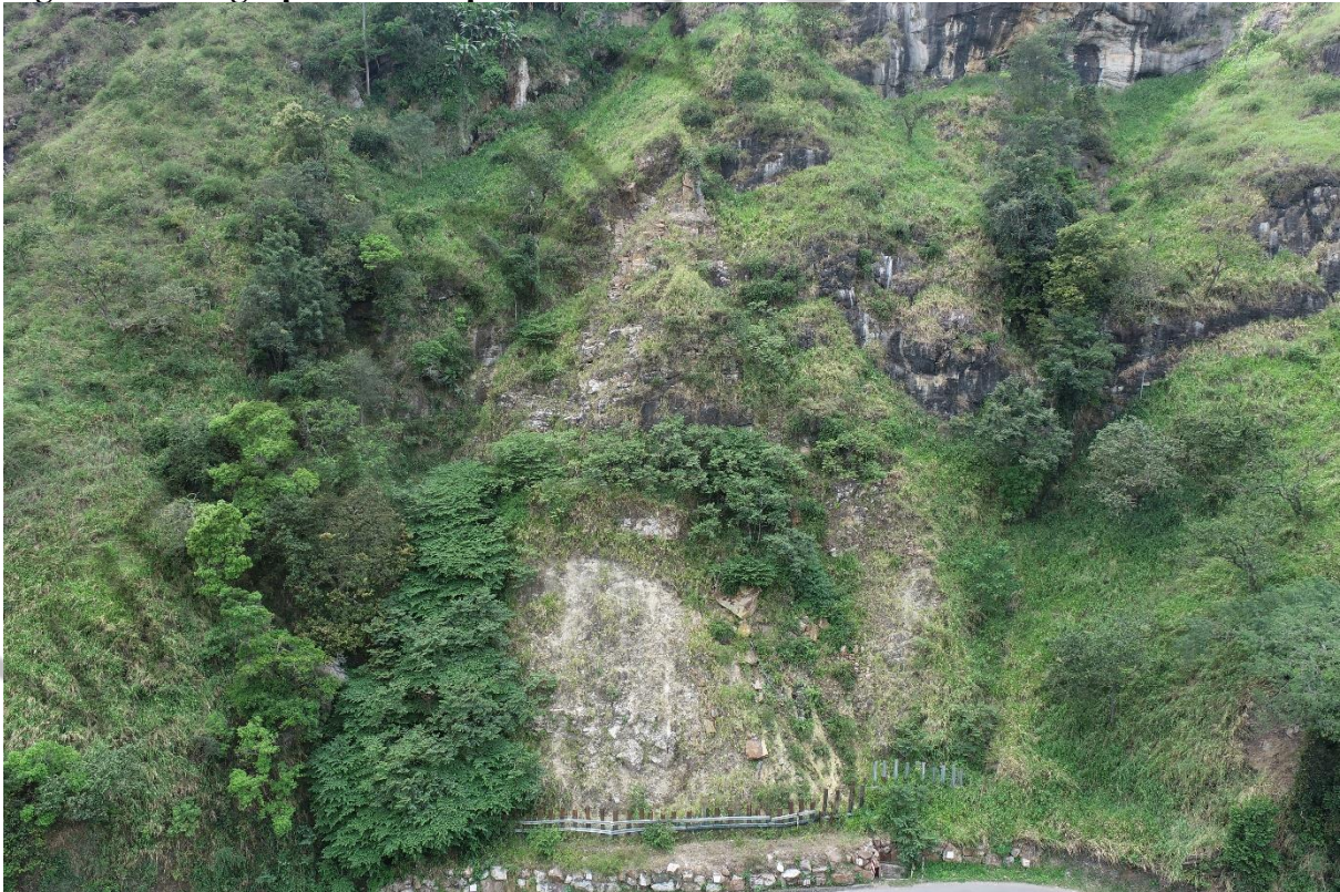
Fig. 3.18 Photograph of the slope with rock debris
