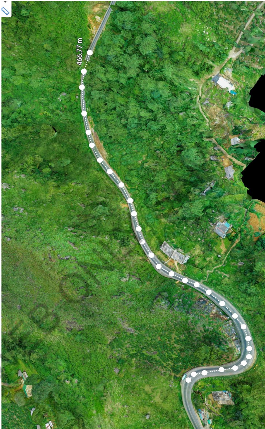
Fig. 3.11 Extent of slope to be rectified
