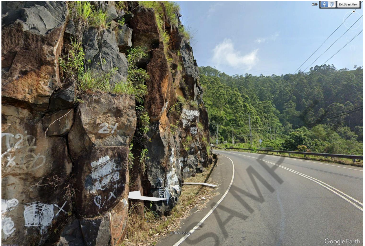
Fig. 3.9 Photograph of the fractured rock slope
