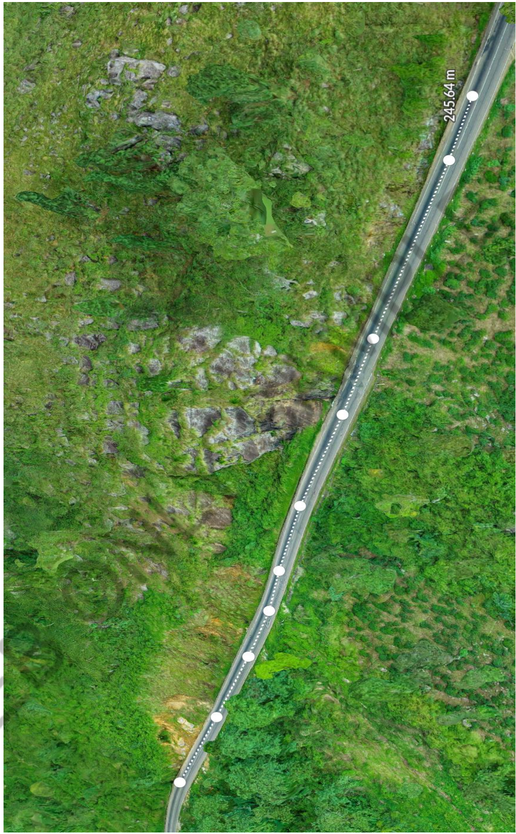
Fig. 3.15 Extent of slope to be rectified
