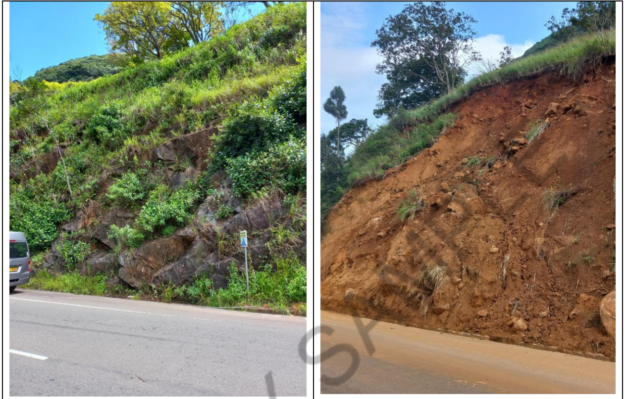
Fig 3.16: View of the unstable rock fragment between culvert No 38/8to 39/9.
