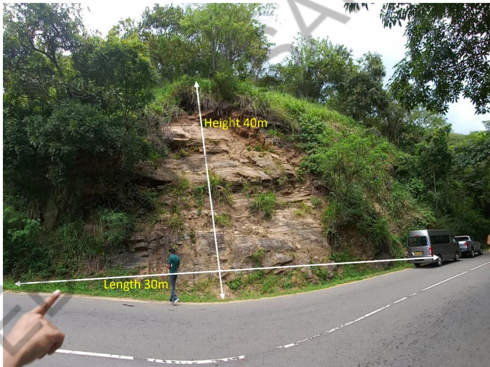
Fig 3.9: Extend of slope to be rectified
