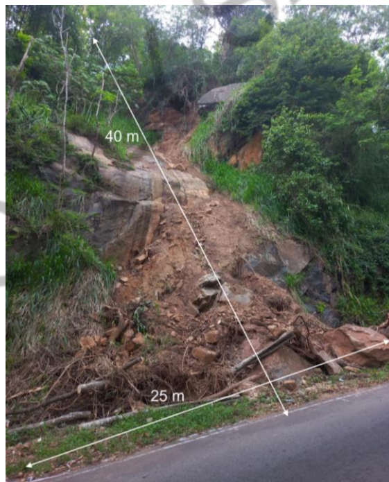
Fig 3.5: Extend of slope to be rectified between 27 km post to 28/1 LHS
