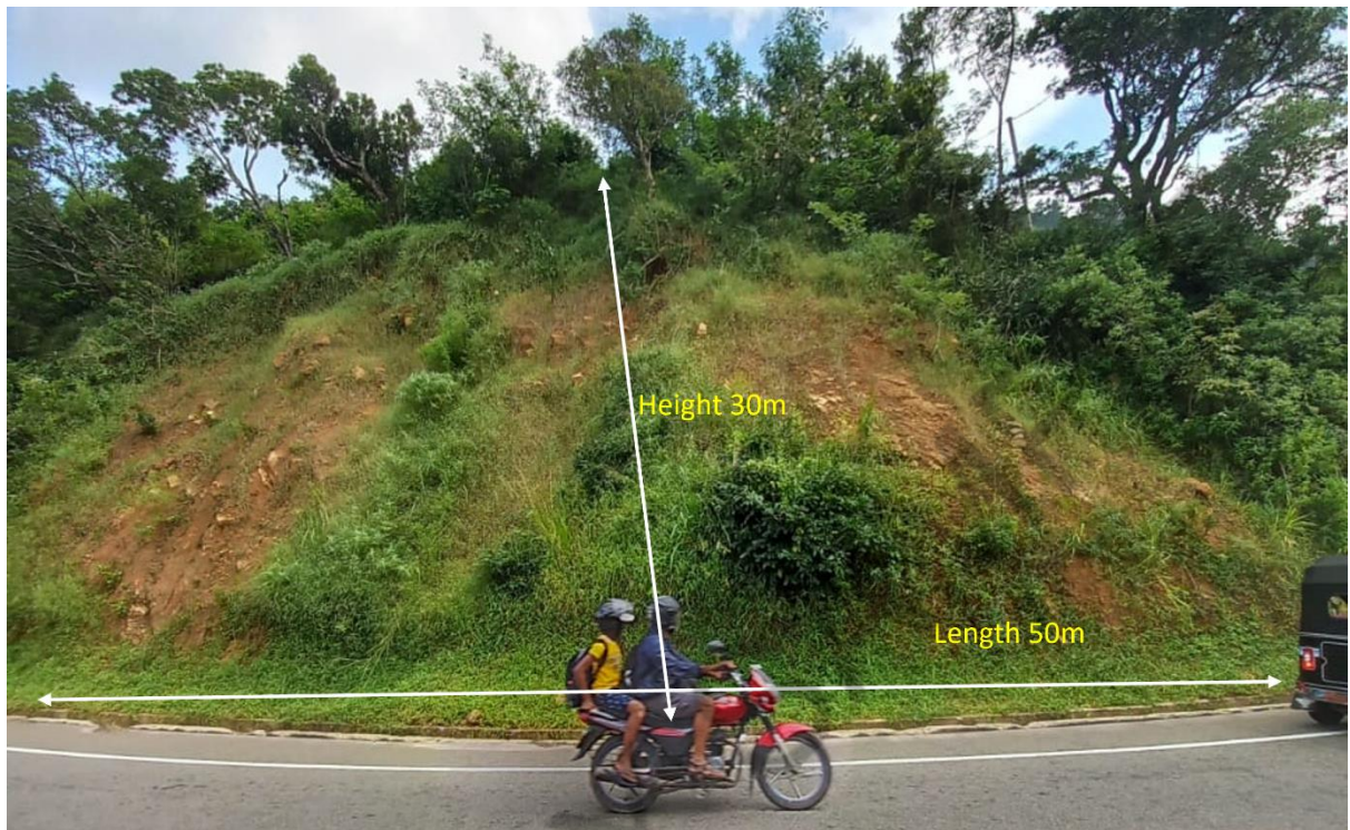
Fig 3.24: Extend of slope to be rectified at 46km to 47/1 RHS
