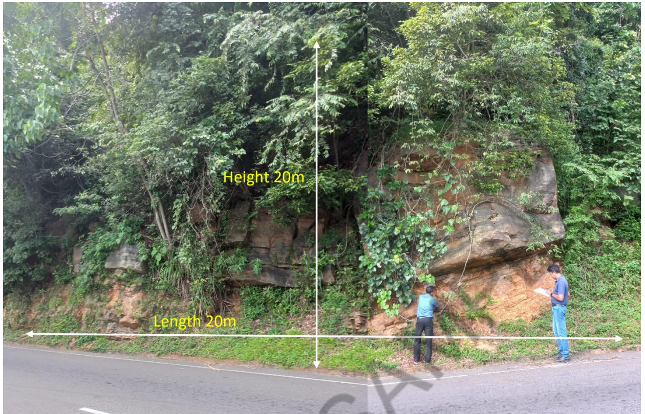
Fig 3.39: Extent of slope to be rectified
