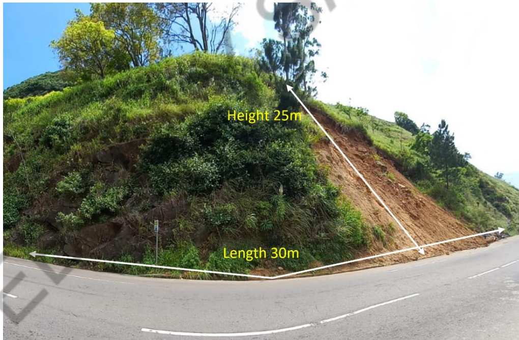
Fig 3.17: Extend of slope to be rectified between culvert No. 38/8 to 38/9
