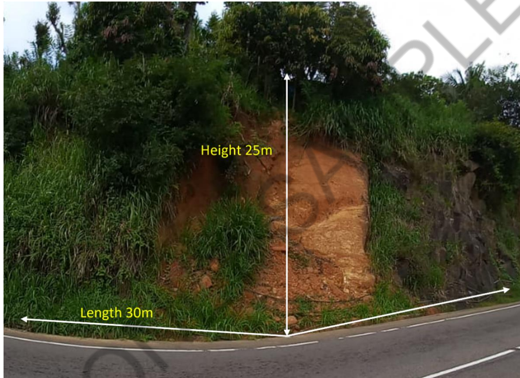
Fig 3.26: Extend of slope to be rectified at 54/5 to 54/6 RHS
