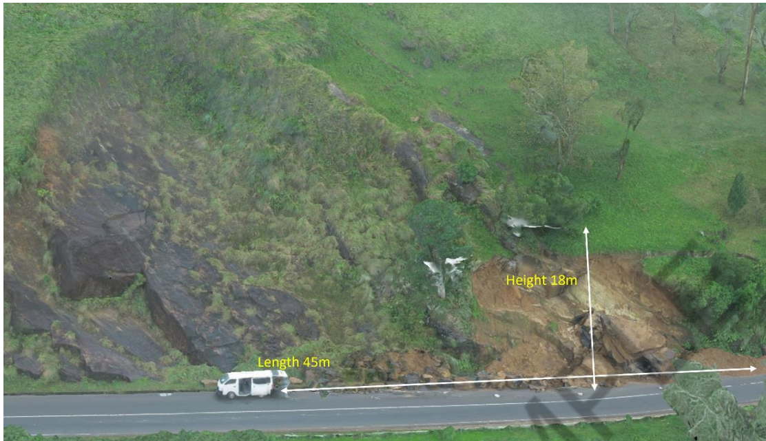
Fig 3.15: Extend of slope to be rectified (Aerial view)
