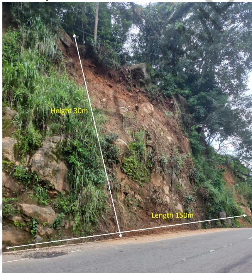
Fig 3.13: Extend of slope to be rectified
