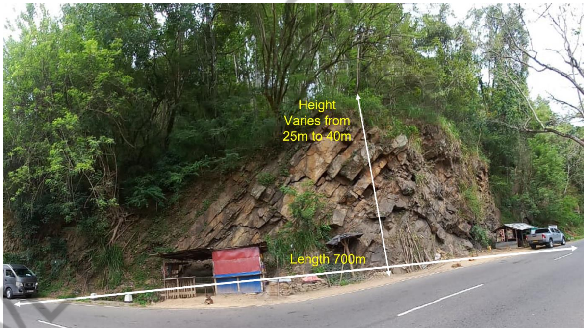
Fig 3.7: Extend of slope to be rectified between 29/3 km to 29/9 LHS
