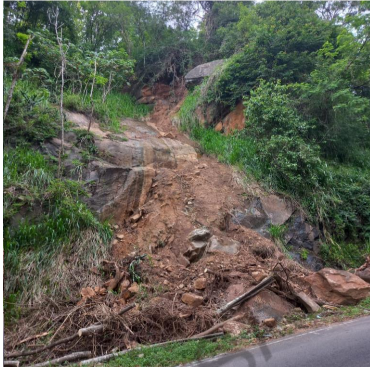
Fig 3.4: View of the collapsed slope and unstable boulders between 27 km post to culvert number 28/1
