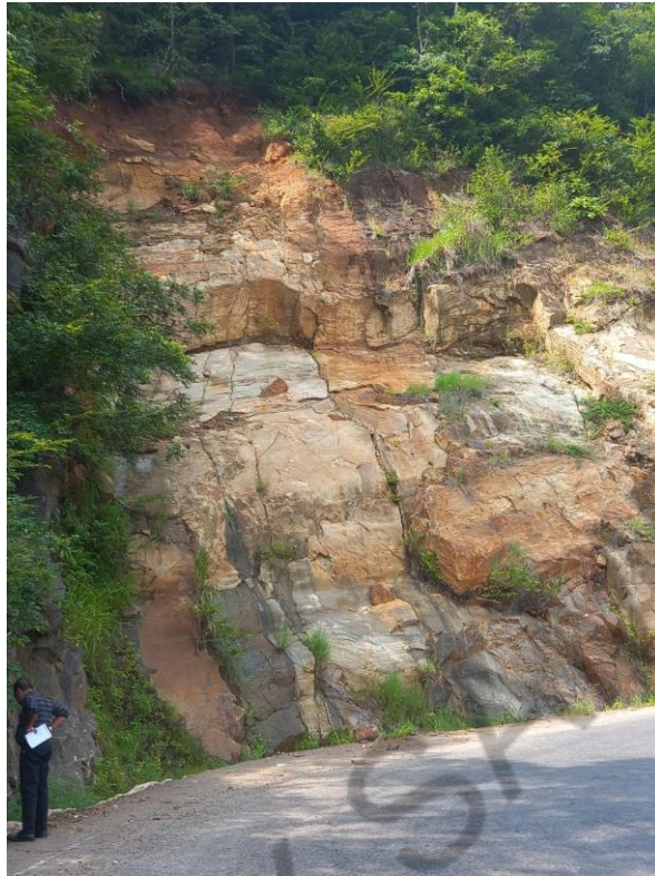
Fig 3.37: View of the unstable boulders at 61km
