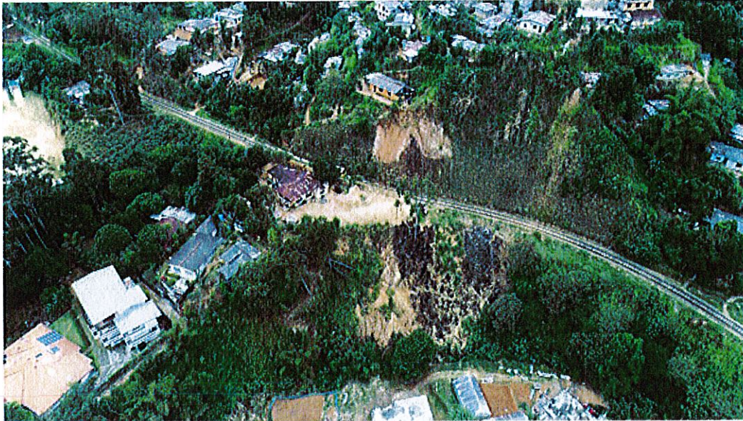
Figure A2.7: Picture of Thapalkanda Landslide Site
