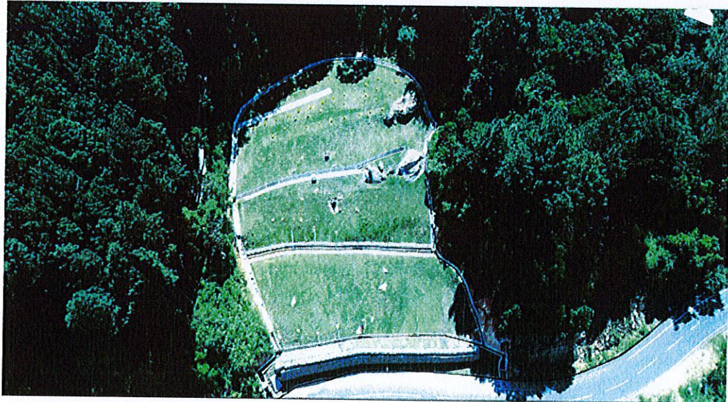
Figure A2.22: Surface Drainage
