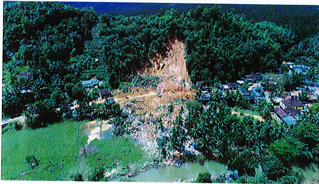
Figure A2.5: Picture of Ayagama Town Landslide Site
