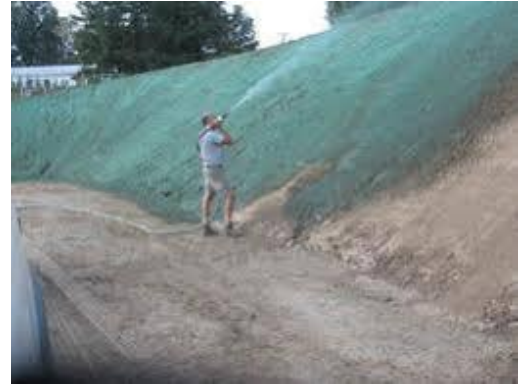
Figure 10: Hydro seeding as a slope erosion control measure
