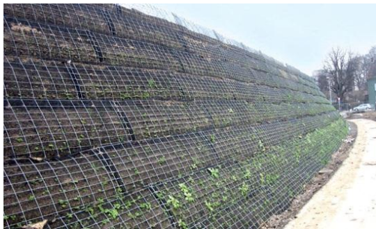
Fig 7: Geogrid application for slope protection: http://www.happho.com/geogrids-
