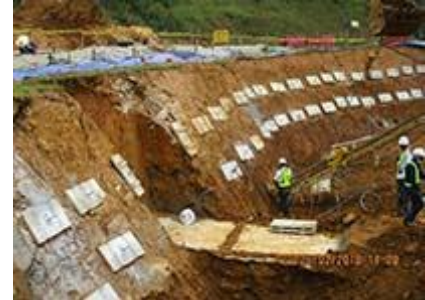
Figure 9: Rock bolting: RDA SL
