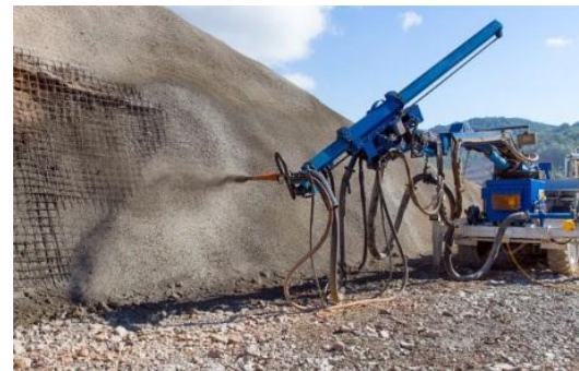
Figure 11: Shotcreting of slopes
