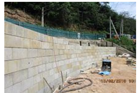
Figure 10 : Retaining wall: RDA SL
