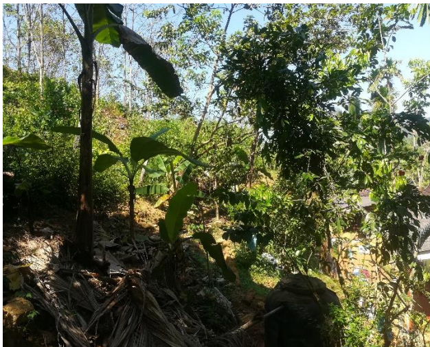
Figure 04 (b) – The unstable slope behind the house located in the landslide prone area
