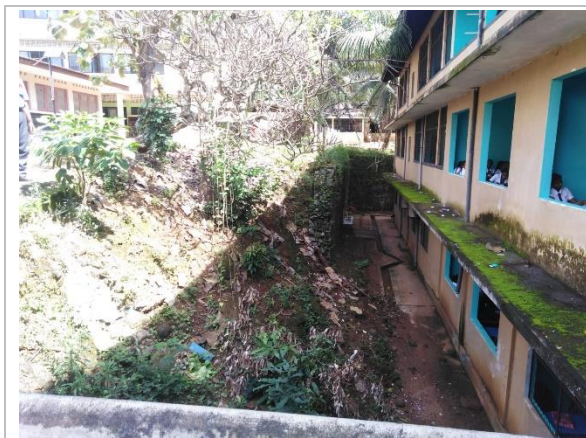
Figure 4a: Unstable slope between chemistry laboratory and three storied building of grade 8
