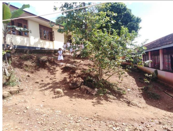
Figure 4c: Slope section between O/L laboratory building and grade 6 single storied building
