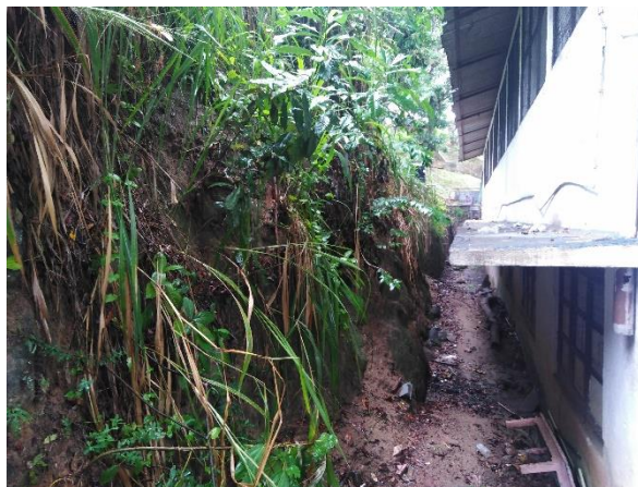
Figure 4c: Slope section behind the Art building (L3)
