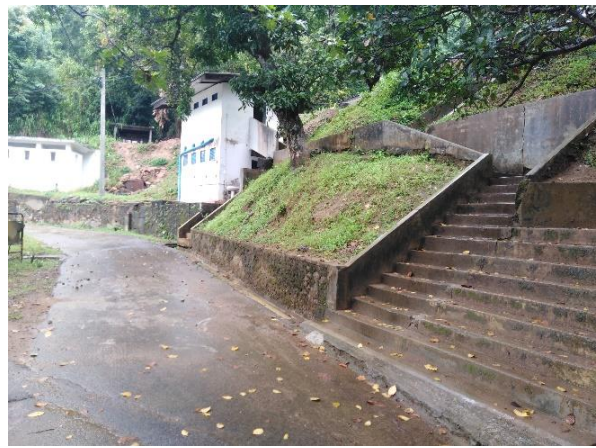
Figure 4f: Stairways near to block C boys showers No.2 (L6)
