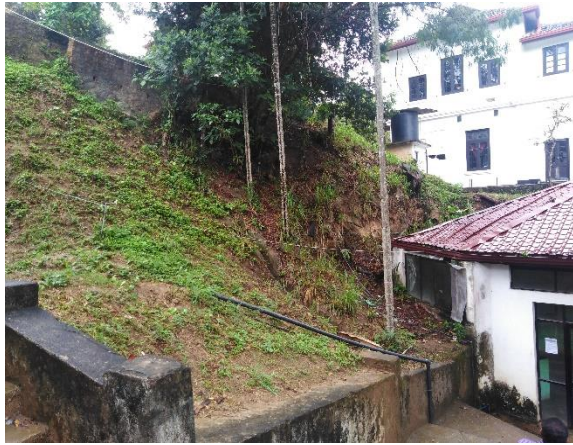
Figure 4g: Land section between hostel and old canteen (L7)
