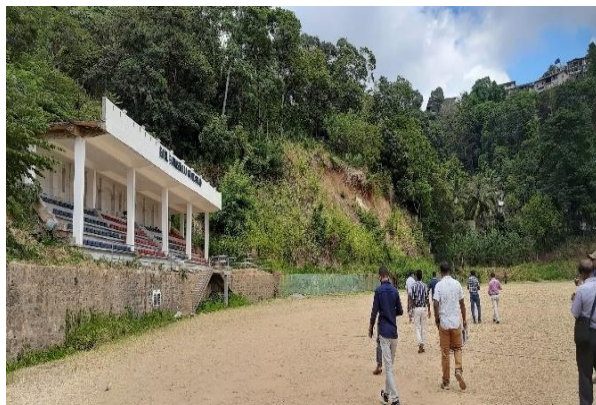
Figure 4J: Slope near the pavilion area (L10)
