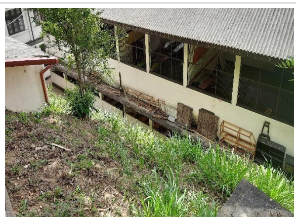
Figure 4b: Infront of the commerce building (RHS of sanitary facility) (L2)
