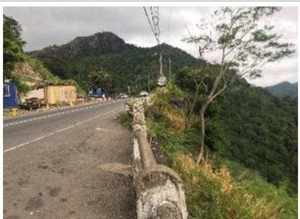
Figure 7b: Down slope of the mitigation site
