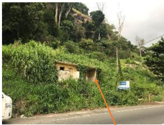
Figure 7c: Damaged toilet compound
