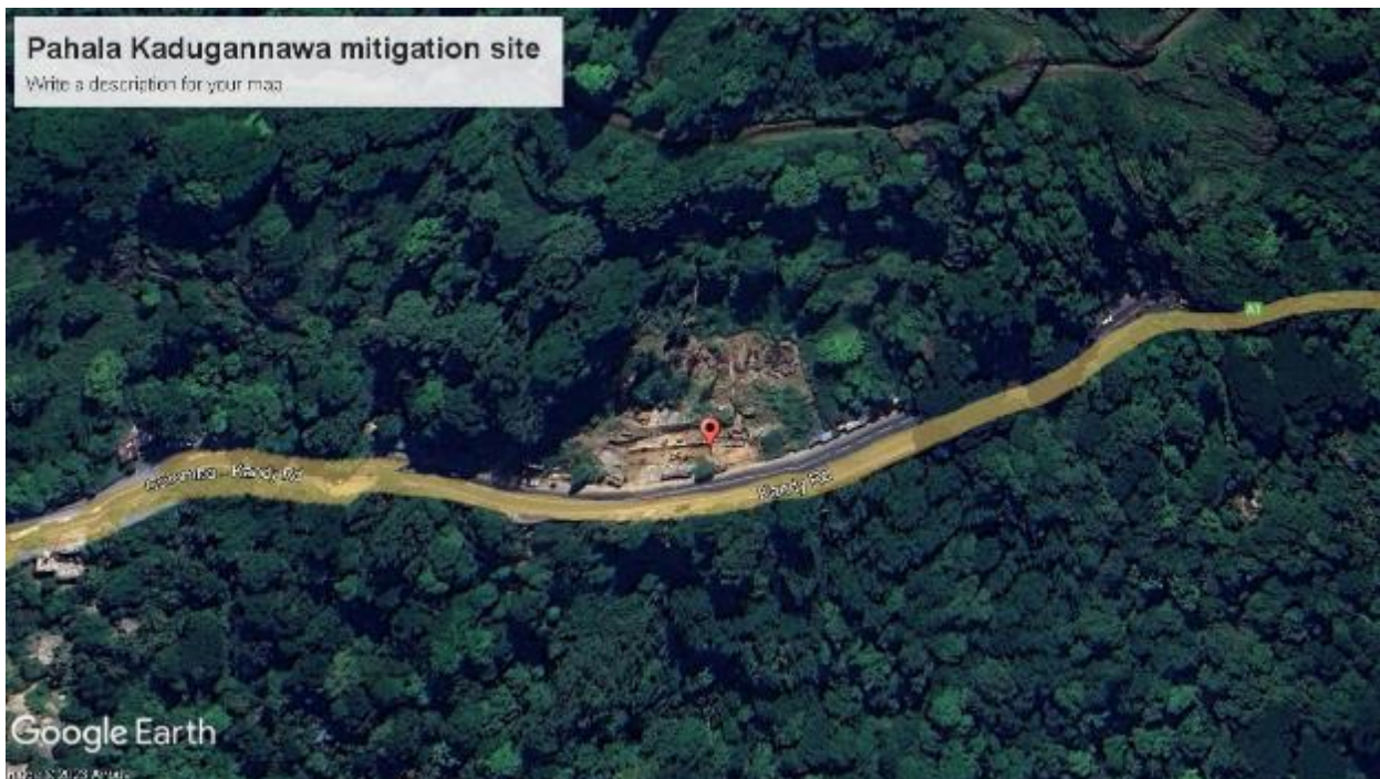
Figure 2: Google image of the proposed landslide mitigation site, the surrounding environmental features and service infrastructure.
