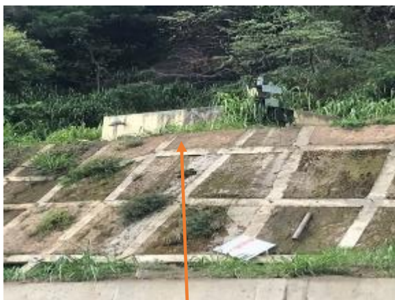
Figure 7d: Water tank
